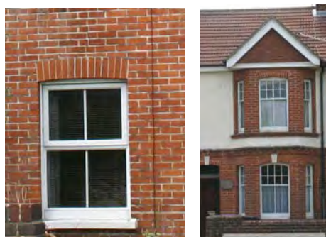
Arched brick headers and flat stone or brick headers are common in the area. Bay windows could be used on key buildings.
